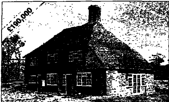
KENT: Idenborough, East Brabourne, Near Ashford. Secluded Grade II listed 16th-century cottage in need of updating, in an acre of land at the foot of the North Downs. Four bedrooms, bathroom, three reception rooms and kitchen. About £190,000 (Calcult Maclean, 01233 812050)
